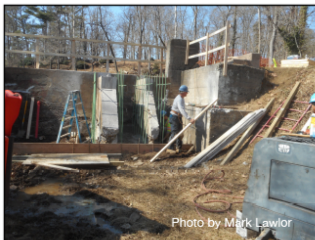
Photo 2 Creating the forms on the Dam. The two north buttresses became one large buttress.
