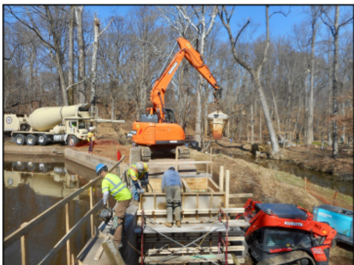
Photo 3 Concrete in the bucket about to be poured into the forms.
