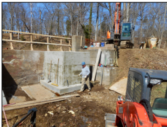
Photo 4 The finished concrete form on the dam.
